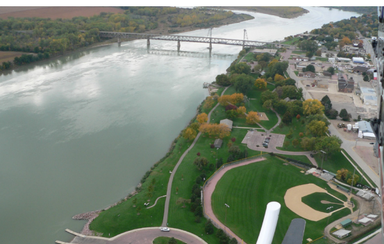
MERIDIAN BRIDGE PROJECT, SD AND NE, A SECTION 106 SUCCESS STORY (NPS)
