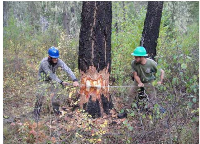
Photos: From left, two log protective weirs with revegetated terrace shown in between; fire-killed trees located along the site were felled and used as weir logs and terrace support elements (photos courtesy USFS)
