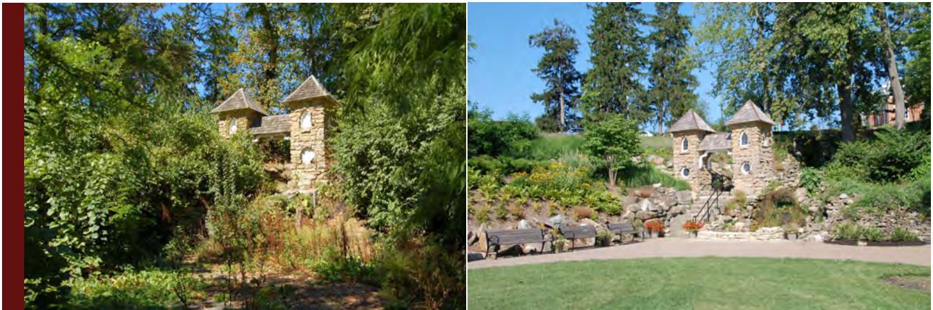
Photos: Grotto gate towers, before (2010) and after restoration (2014) (photos courtesy American Veterans Heritage Center)
