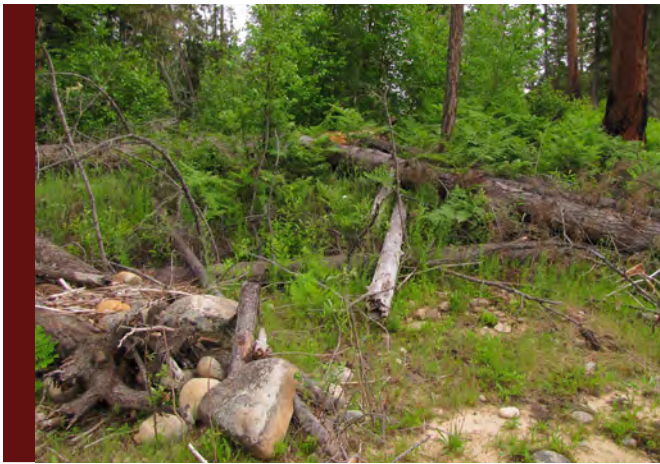
Photos: From left, two log protective weirs with revegetated terrace shown in between; fire-killed trees located along the site were felled and used as weir logs and terrace support elements (photos courtesy USFS)
