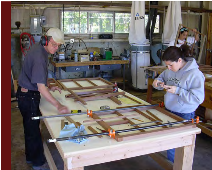
Photos: Above, historic windows were repaired in a training workshop in 2003; Right, lime stucco repair and repair of wood moldings (photos courtesy MCB Camp Pendleton)
