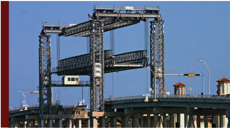
Above: Temporary bridge with lift; bridge for boat traffic adjacent to the historic bridge. © L. Barnwell Right: Bridge of Lions © Paul Brennan
