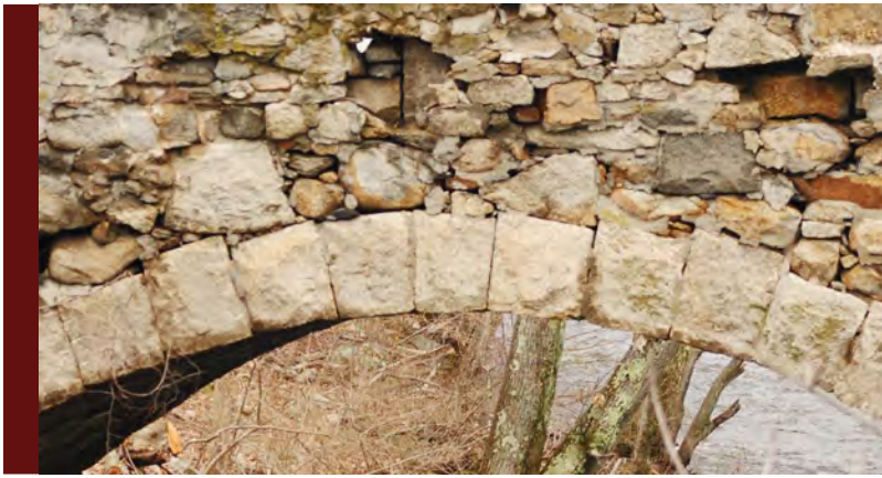
Photos: Left, detail of degraded spandrel wall masonry before restoration; Right, stone arch exposed after road bed stripping and systematic deconstruction of spandrel masonry; almost complete in summer 2017 (photos courtesy RI SHPO)
