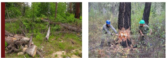
Photos: From left, two log protective weirs with revegetated terrace shown in between; fire-killed trees located along the site were felled and used as weir logs and terrace support elements (photos courtesy USFS)
