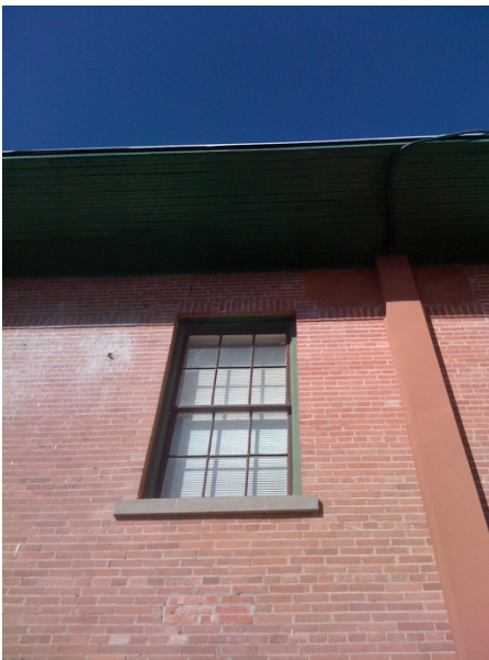
Building 115 – Window & Eave
