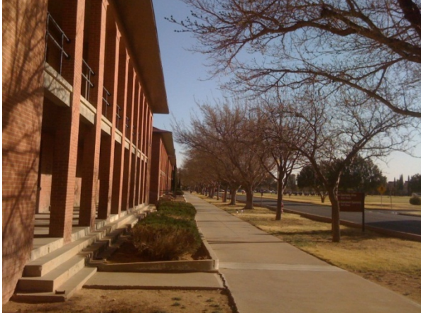
Building 115 – Front on Pershing Road
