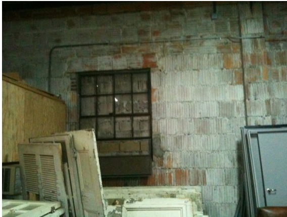
Building 61: Clay Tile Wall
