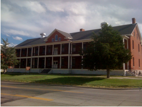
Building 222 - Wing at Rear
