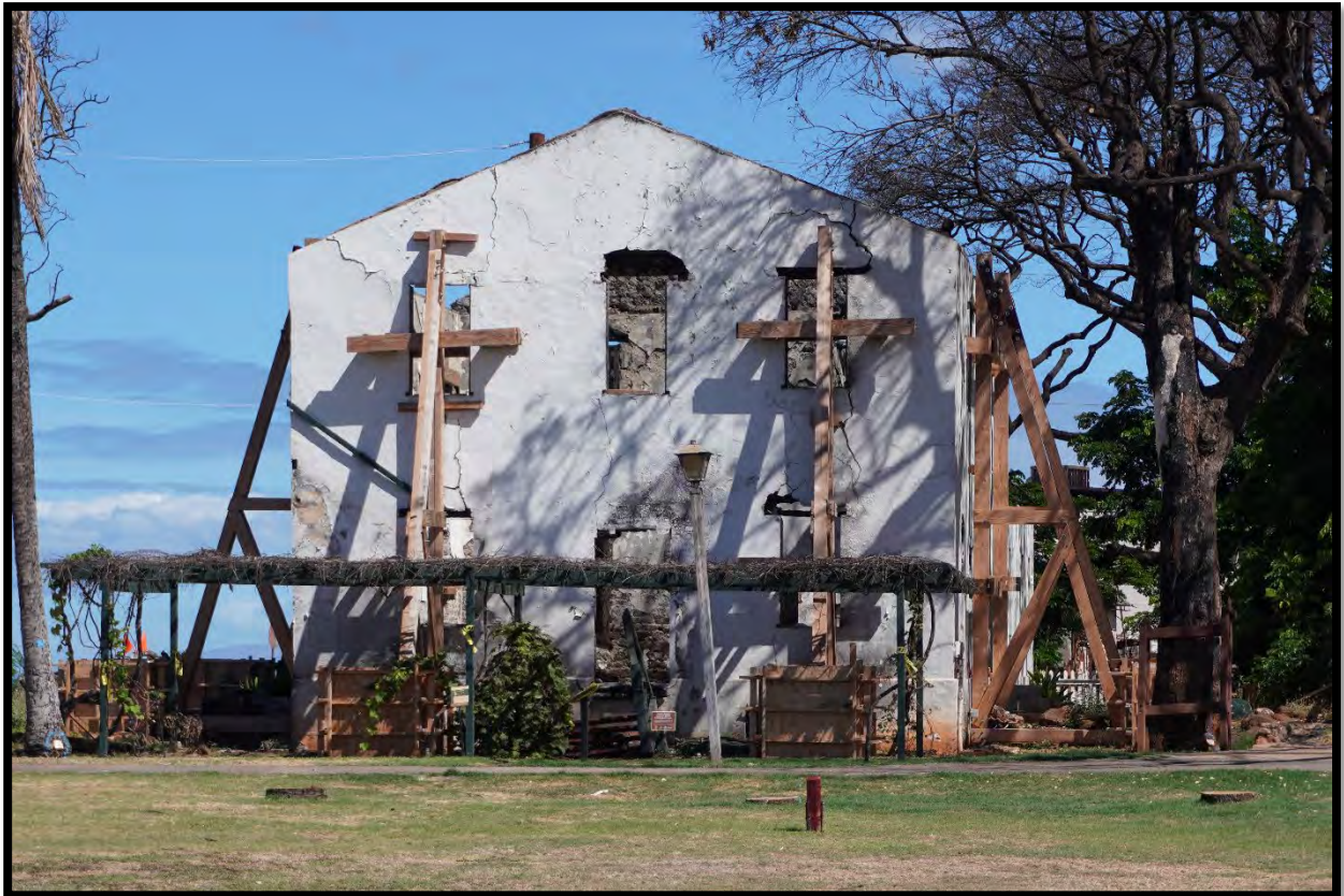
Figure 9. South façade of the Baldwin House showing fire damage and shoring. NPS Photo taken July 29, 2024.
