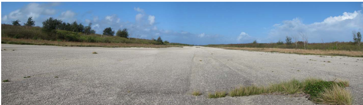
Character defining view down Runway Able, facing west (CLR, 3-27).
