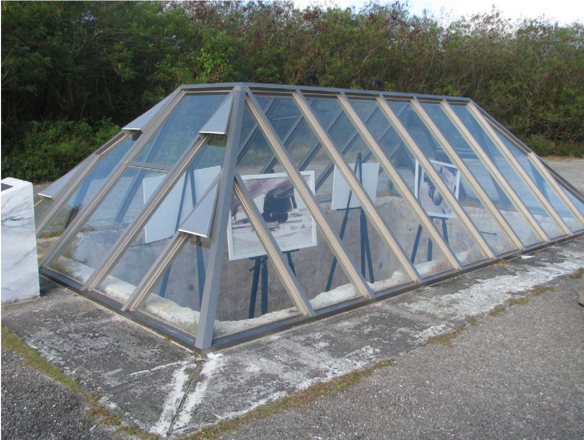
Atomic Bomb Loading Pit with non-historic protective glass structure ( CLR , 3-43).
