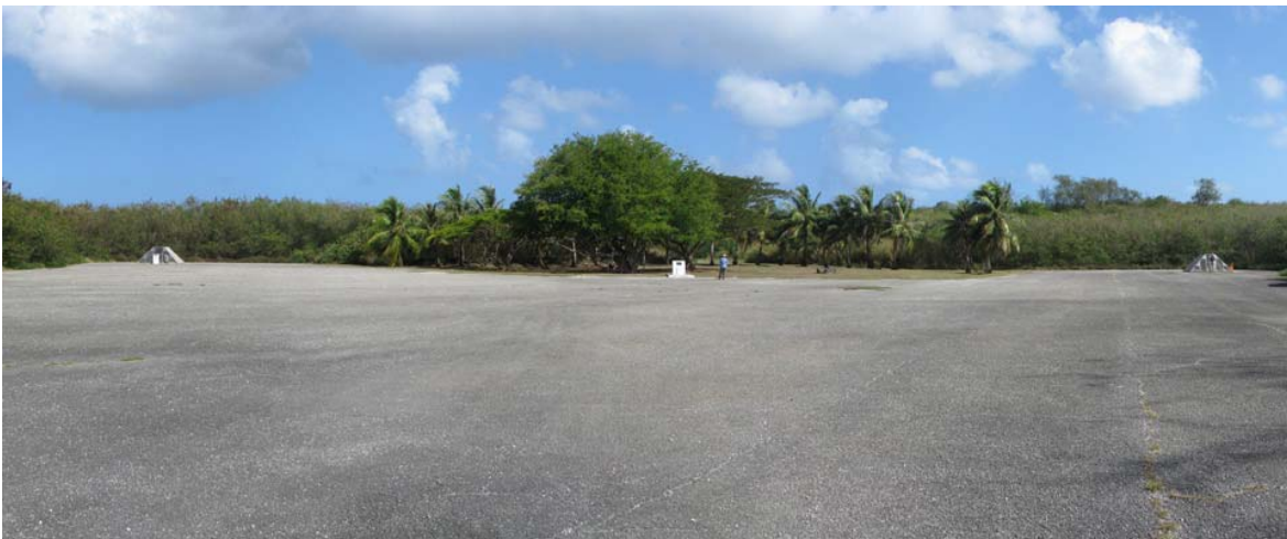
Atomic bomb loading apron. Loading pit protective glass structures are visible on the right and left. The NHL marker is also visible in the center, backed by an area of non-historic ornamental plantings ( CLR , 4-19).
