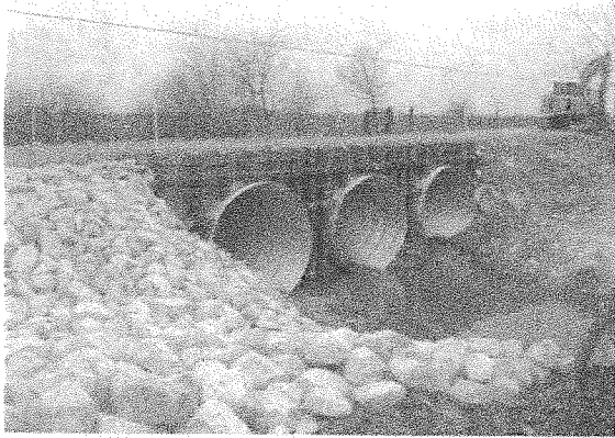
Figure 7 ~ Road Crossing: Timber abutment with rock chute
