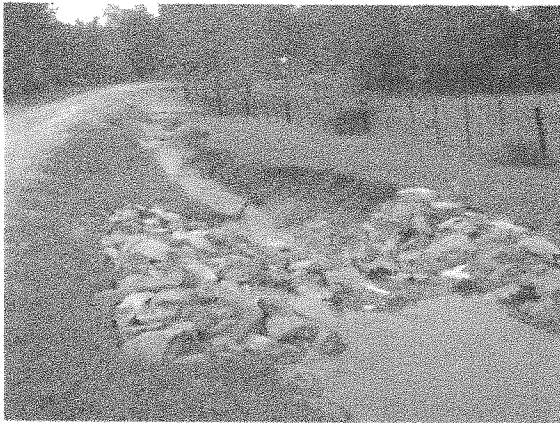
Figure 9 ~ Ditch Stabilization: Rock riprap check dams
