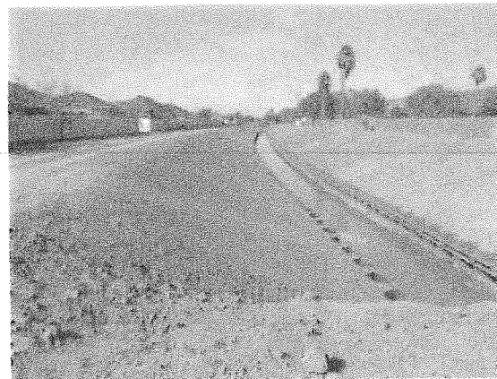
Figure 16 – Drainage Ditch Stabilization: Steel sheet piling and bank shaping
