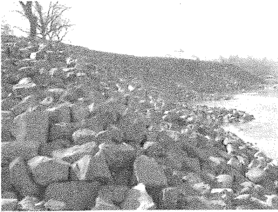
Figure 1 – Streambank Protection: Rock riprap armor with rock weirs
