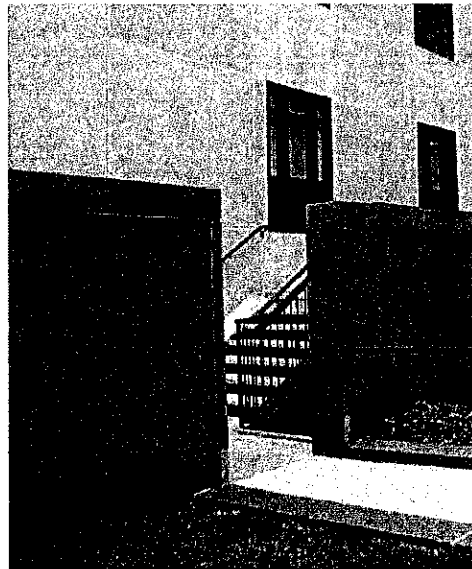
View of proposed areaway wall after access has been created. Removed granite to be salvaged and stored.
