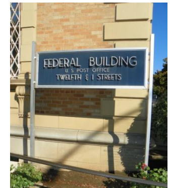
Existing Federal Building U S Post Office sign. To be removed.
