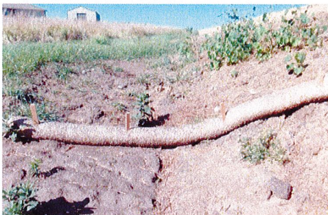
Erosion control: wattle
