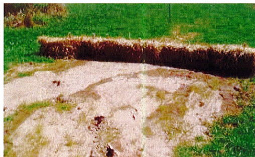
Erosion control: straw bales
