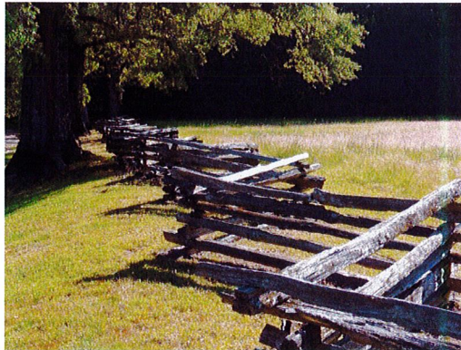
Zig-Zag Split Rail Fencing
