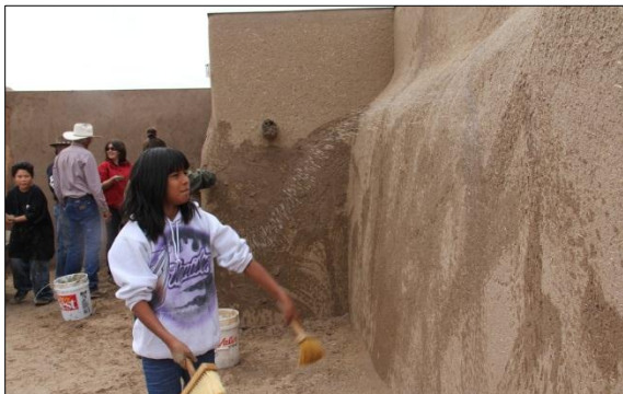
A mud plastering workshop as part of the Owe'neh Bupingeh Preservation Project in New Mexico where tribal members, including many young people, repaired and enhanced housing within the pueblo. Photo by Tania Hammidi
