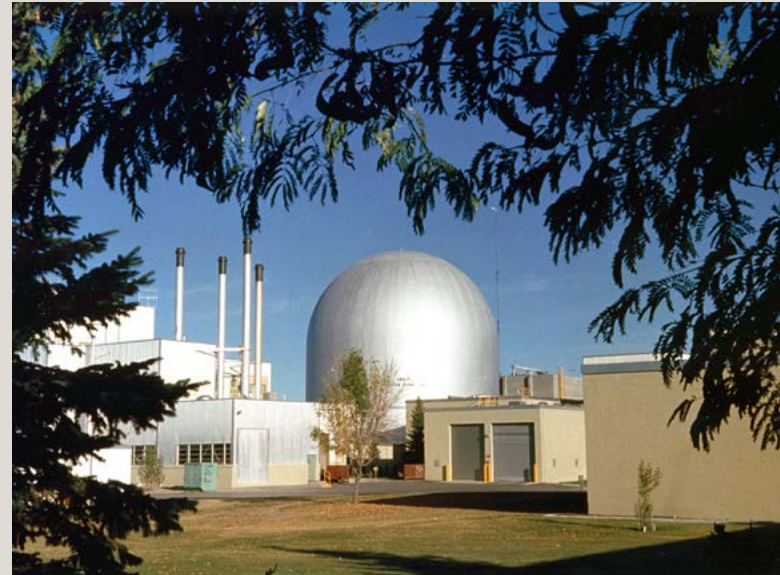
EBR-II is eligible for the National Register and was spared from demolition through repurposing as a microreactor test bed facility. (Idaho National Laboratory)
