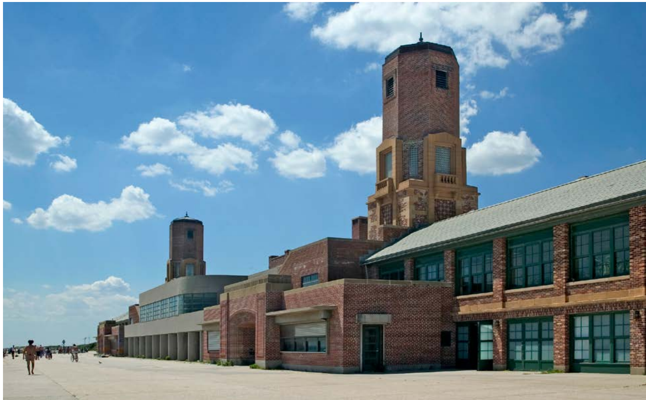
Restoration work on the 1930s Jacob Riis Bathhouse within Gateway National Recreation Area has addressed hurricane and erosion damage to the property from Hurricane Sandy in 2017. (NPS)
