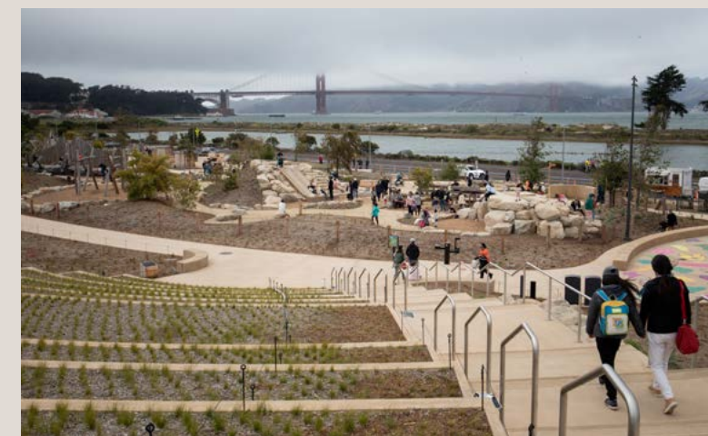
Top: Tunnel Tops nearing completion (James Corner Field Operations)
