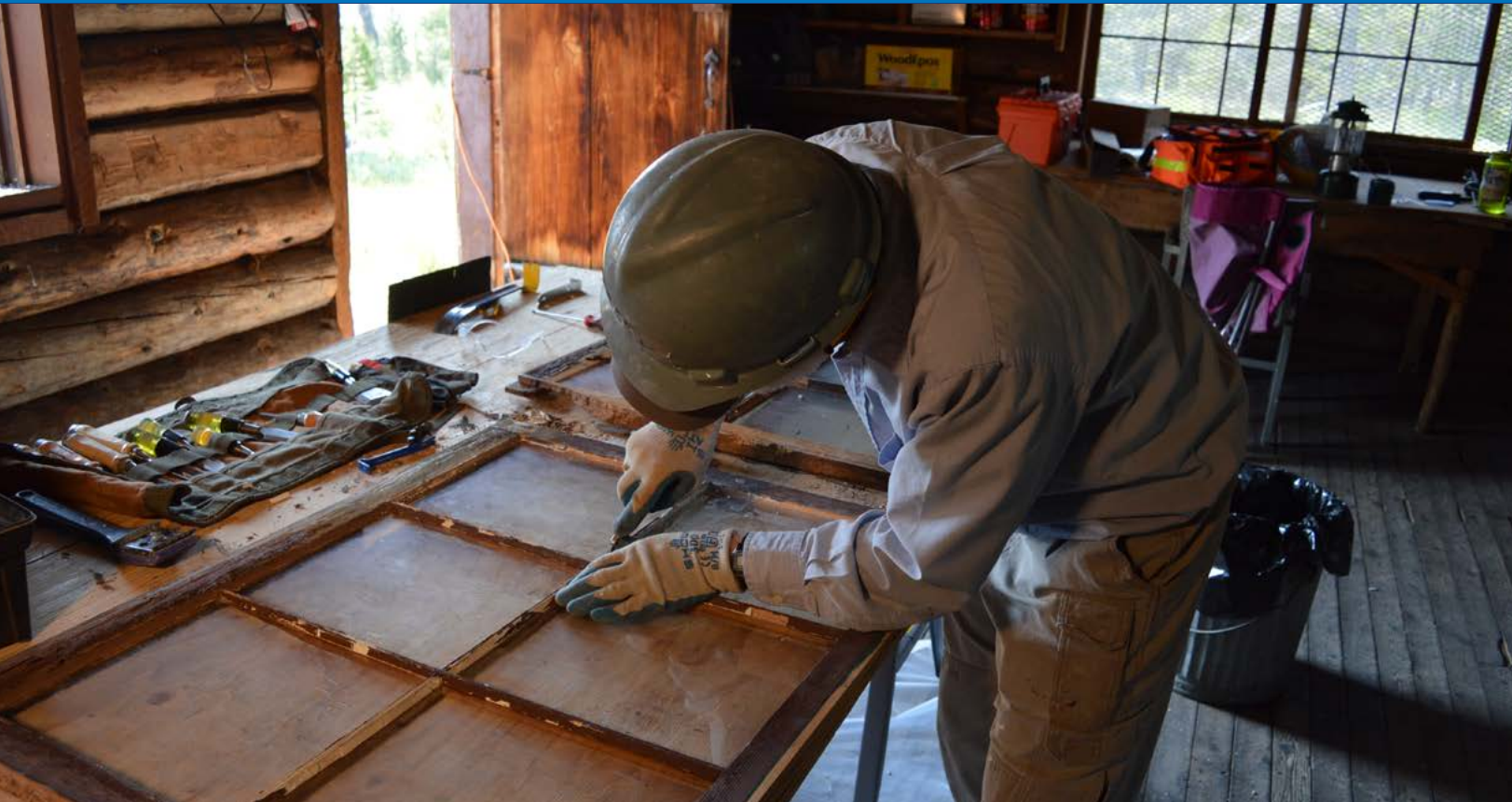
A HistoriCorps volunteer glazes windows as part of the restoration of Corral Park Cabin within the Arapaho and Roosevelt National Forests and Pawnee National Grassland. (Erica Bradley/USFS)
