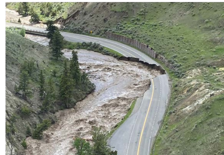
Unprecedented amounts of rainfall combined with snowmelt caused severe damage to infrastructure including the north entrance road at Yellowstone National Park in June 2022. (Doug Kraus/NPS)
