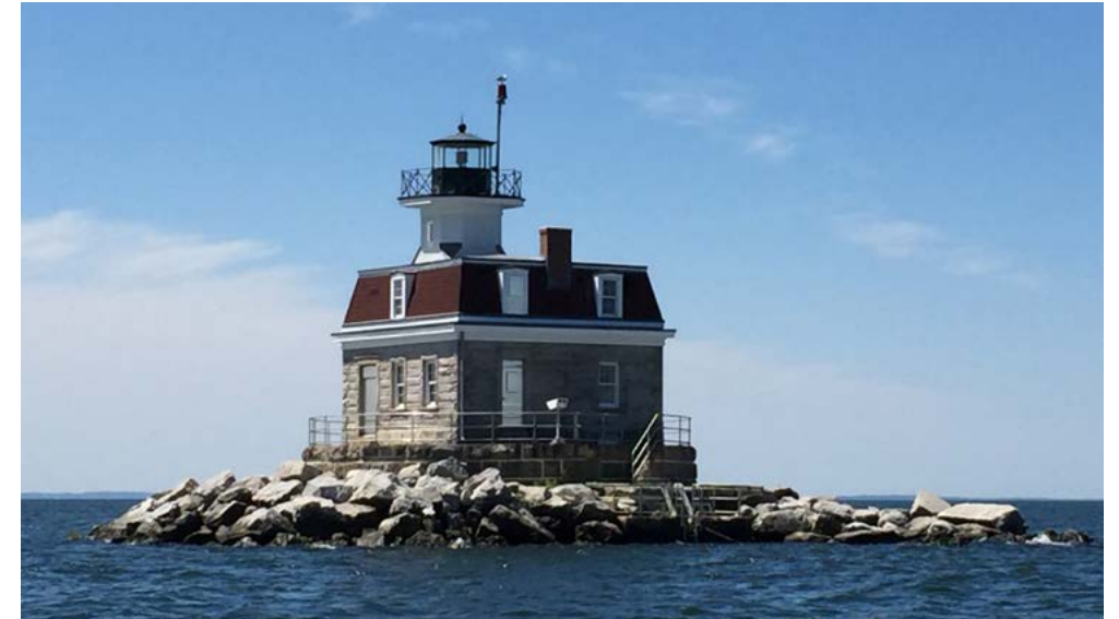
Under the NHLPA, GSA, NPS, and USCG work together to find new stewards for decommissioned historic lighthouses. GSA sold the Penfield Reef Light in Long Island Sound with preservation covenants in 2022. (GSA)
