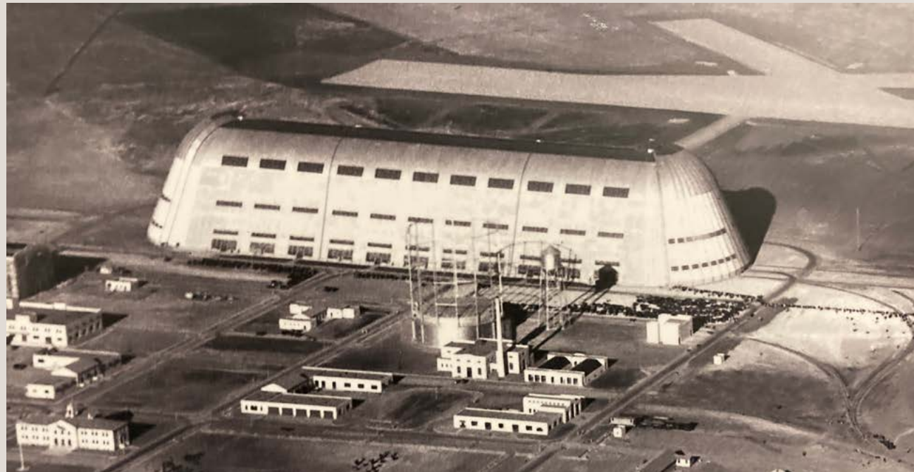
Historic photo of the completed Hangar 1 (Moffett Field Historical Society Museum)
