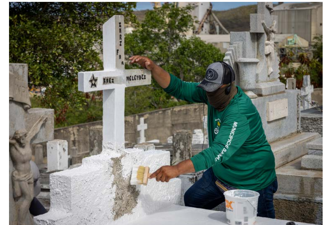
An NCPTT program participant applies whitewash to a gravestone at the Cementerio Católico San Vicente de Paul, Ponce, PR. (James Barry/NPS)
