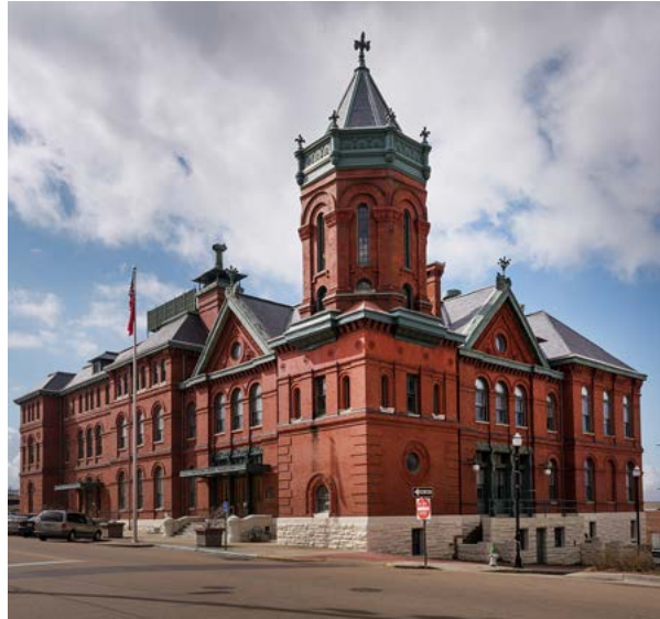
The Mississippi River Commission building, Vicksburg, MS. Planned repairs to the roof, walls, windows, and interior building systems will restore the building's physical integrity, improve safety, reduce operating costs, and extend its service life for another 125 years. (Carol M. Highsmith Photography, Inc./GSA)
