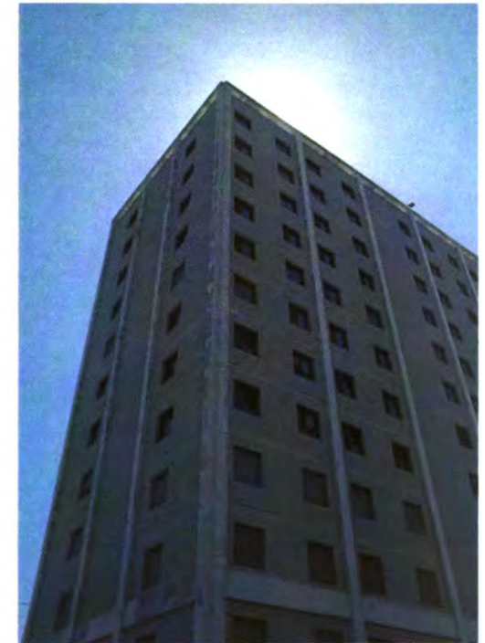
Lockefield Garden Apartments. A net energy-investment advantage over an equivalent new complex for more than 50 years.
