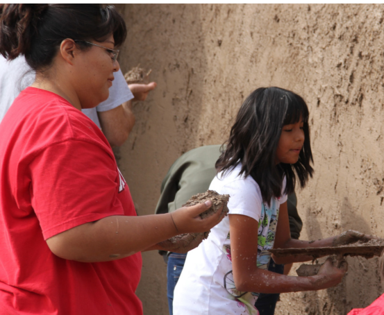
MUD PLASTERING WORKSHOP, OWE'NEH BUPINGEH PRESERVATION PROJECT, NM (TANIA HAMMIDI)
