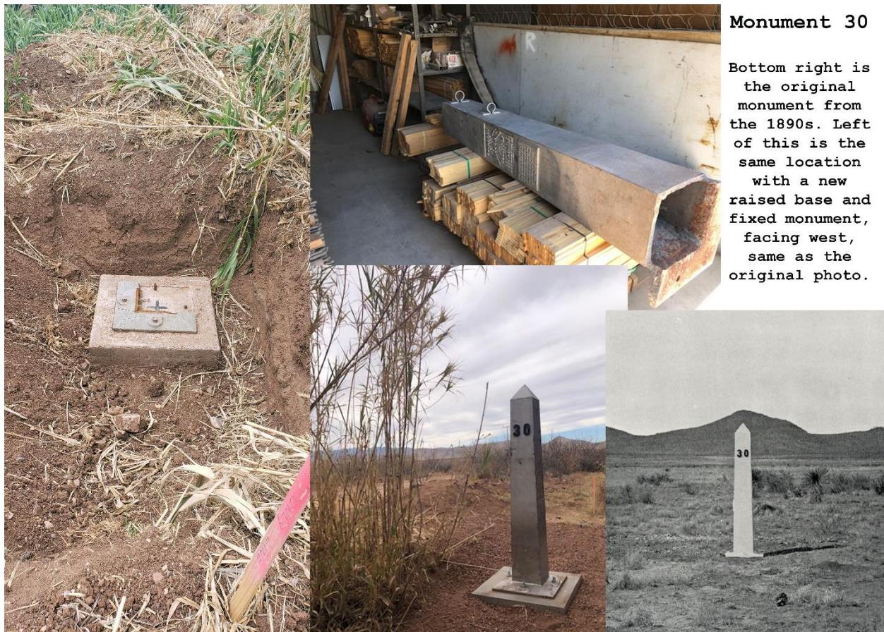
Figure 8: Monument 30 from when established, broken, fixed, and replaced on new raised concrete base.
