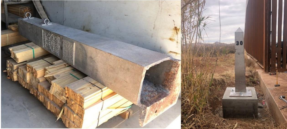
Figure 1: Monument 30 after removal when base was broken and reinstallation after base was fixed and concrete base height was extended.
