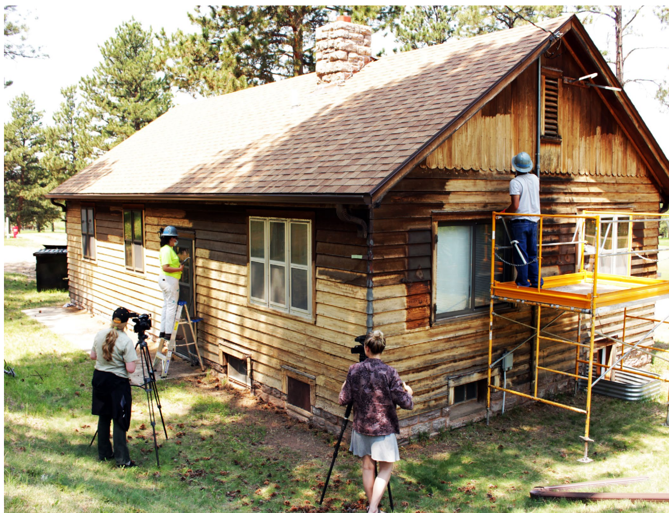
Videographers capture the progress of Boxelder and Pine Ridge Job Corps facilities maintenance, painting, and carpentry students as they restore structures at the Tepee Work Center on the Black Hills National Forest. The students repaired siding and shutters; removed deteriorated, oil-based coatings from the wooden structures; and, to prevent further deterioration, recoated the wood with a Heritage Natural Finish. USDA Forest Service photo by Scott Jacobson.
