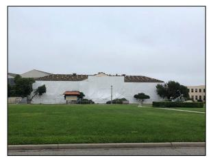
Figure 4-6. Exterior asbestos containment at Buiding 25.
