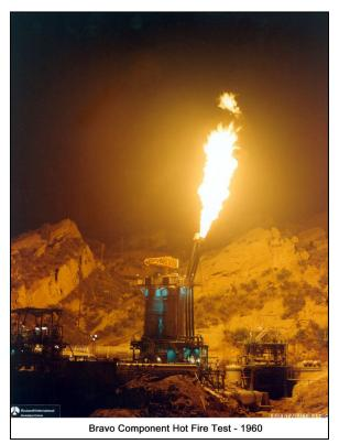
Figure 5-11. 1960 Photo of Bravo Test Stand undergoing a hot fire test.
