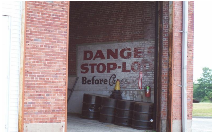
EPA Maintains this c. 1945 Historic Sign in a Maintenance Bay at the Edison Environmental Center as a Link to the Property’s History
