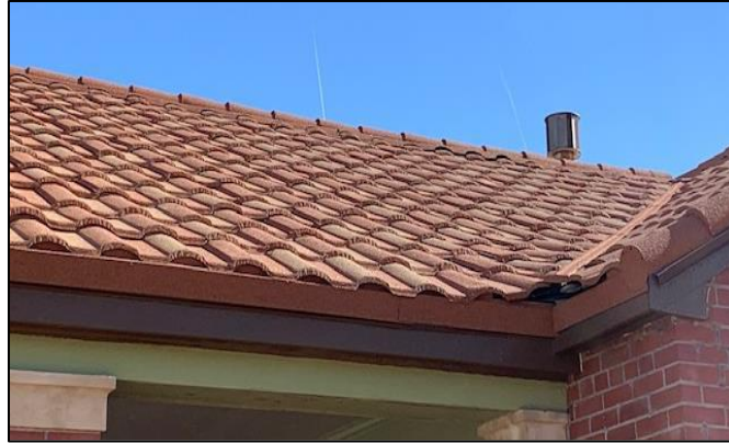
Metal tile roofing on Inter-War Era housing at Fort Bliss.
