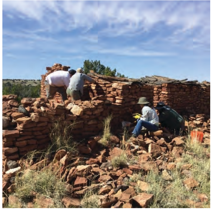
Figure 10. At Red House Pueblo, Coconino National Forest Heritage Professionals work with students and volunteers to repair masonry joints to stabilize the pueblo in hopes that it will stand for another 800 years. (USDA Forest Service photo by Jeremy Haines)
