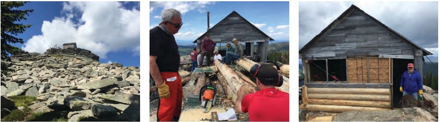
Figure 16. From left to right: view of Skookum Butte Lookout perched atop granite outcrop; volunteers hand-peeling logs to replace deteriorated ones; completed log replacement. (USDA Forest Service photos by Sydney Bacon)
