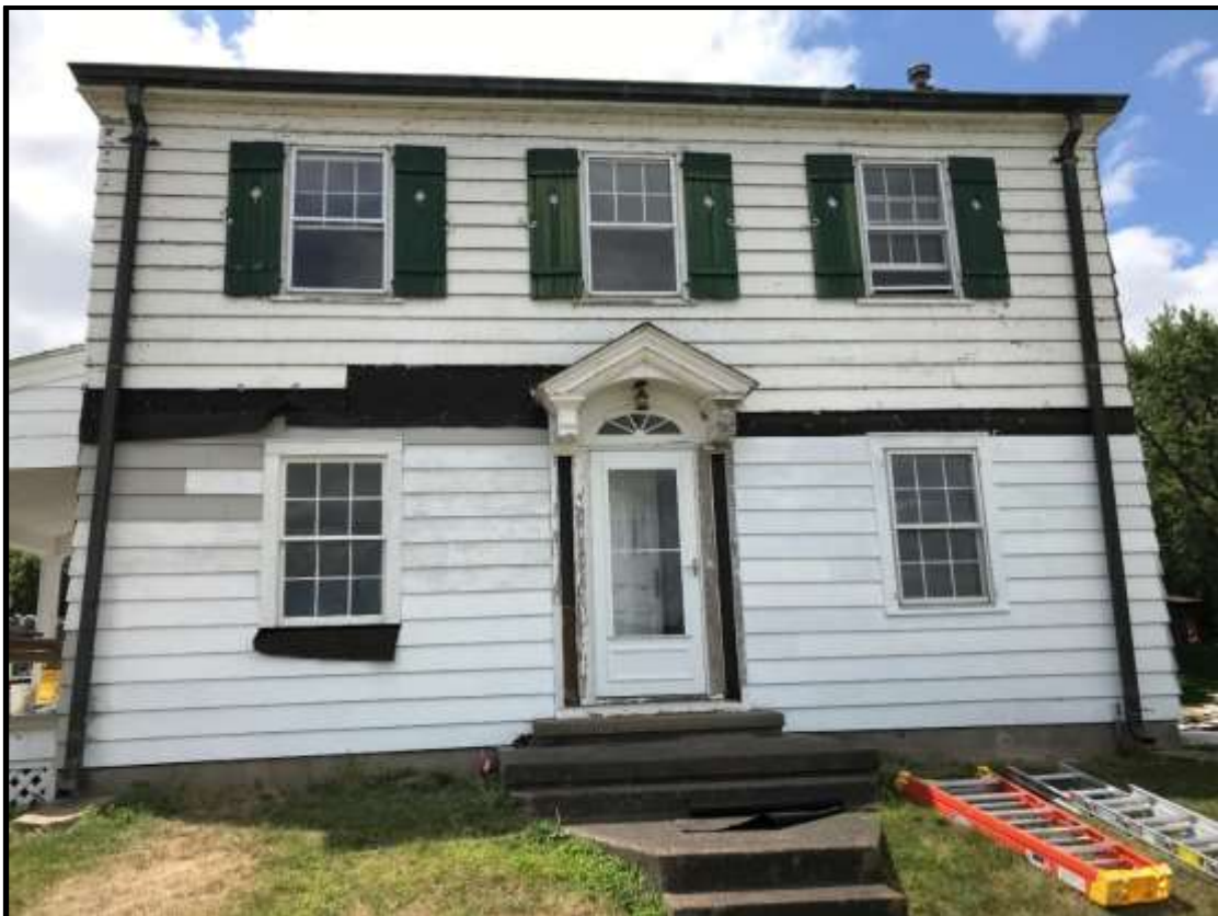
Figure 9: Front of the Lock and Dam 10 Lockmaster house undergoing rehabilitation as
