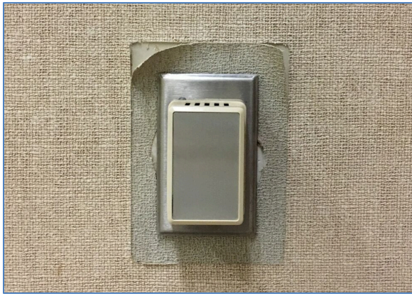
Figure 4-5. Section of original wallpaper that remained intact behind a thermostat cover.
