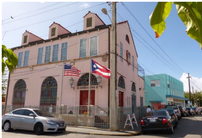
Figure 2: Fajardo Customs House in February 2017. Note altered fenestration and coloring of replacement windows.
