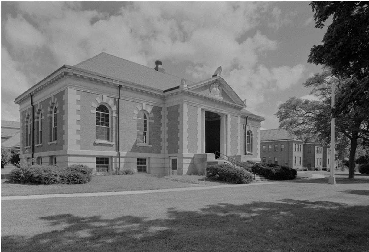
Figure 4 (above): In 2019, VA disposed of Building 48 at the Danville, IL VAMC, the Carnegie Library, with a preservation covenant. It is now property of the Danville Community College (HABS IL-1232-C-5).
