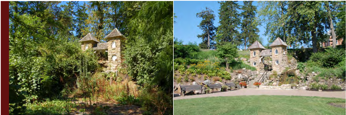
Photos: Grotto gate towers, before (2010) and after restoration (2014) (photos courtesy American Veterans Heritage Center)
