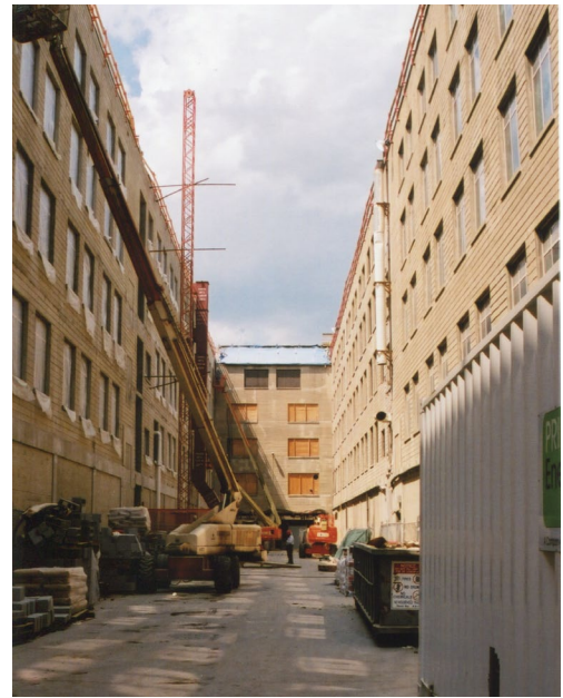
Photos: views of the original and reconstructed sections of the Pentagon
