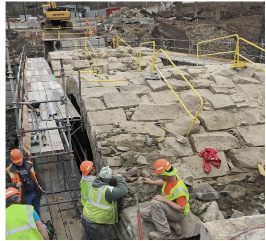
Photos: Left, detail of degraded spandrel wall masonry before restoration; Right, stone arch exposed after road bed stripping and systematic deconstruction of spandrel masonry; almost complete in summer 2017 (photos courtesy RI SHPO)
