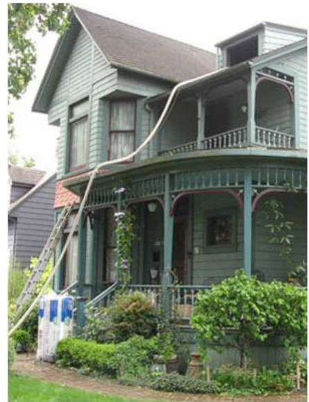
A Department of Energy-funded project in Washington provides insulation for this historic home. (photo courtesy DOE)
