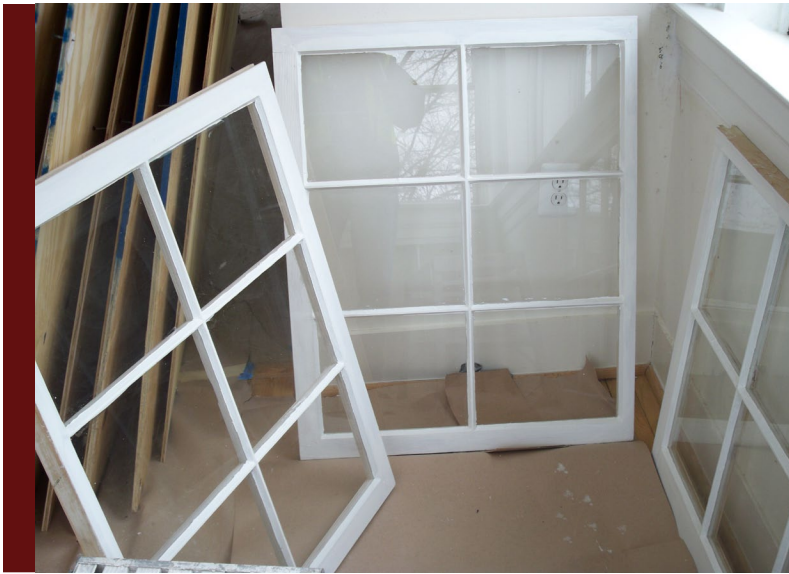
Photos: Above, replacement window installation underway; Right, a worker repairs, abates historic frames on a house in Fort Belvoir Historic District. (photos courtesy U.S.Army)
