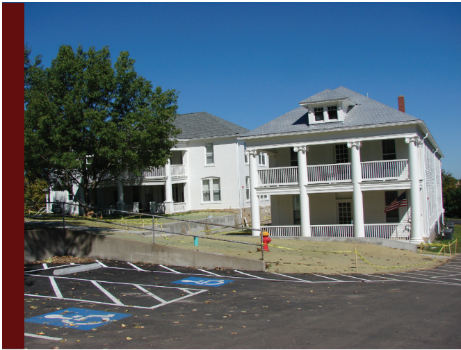
Photos: Left, Buildings 34, 76; Right, Building 76 hallway corridor after renovation (photos courtesy VA)
