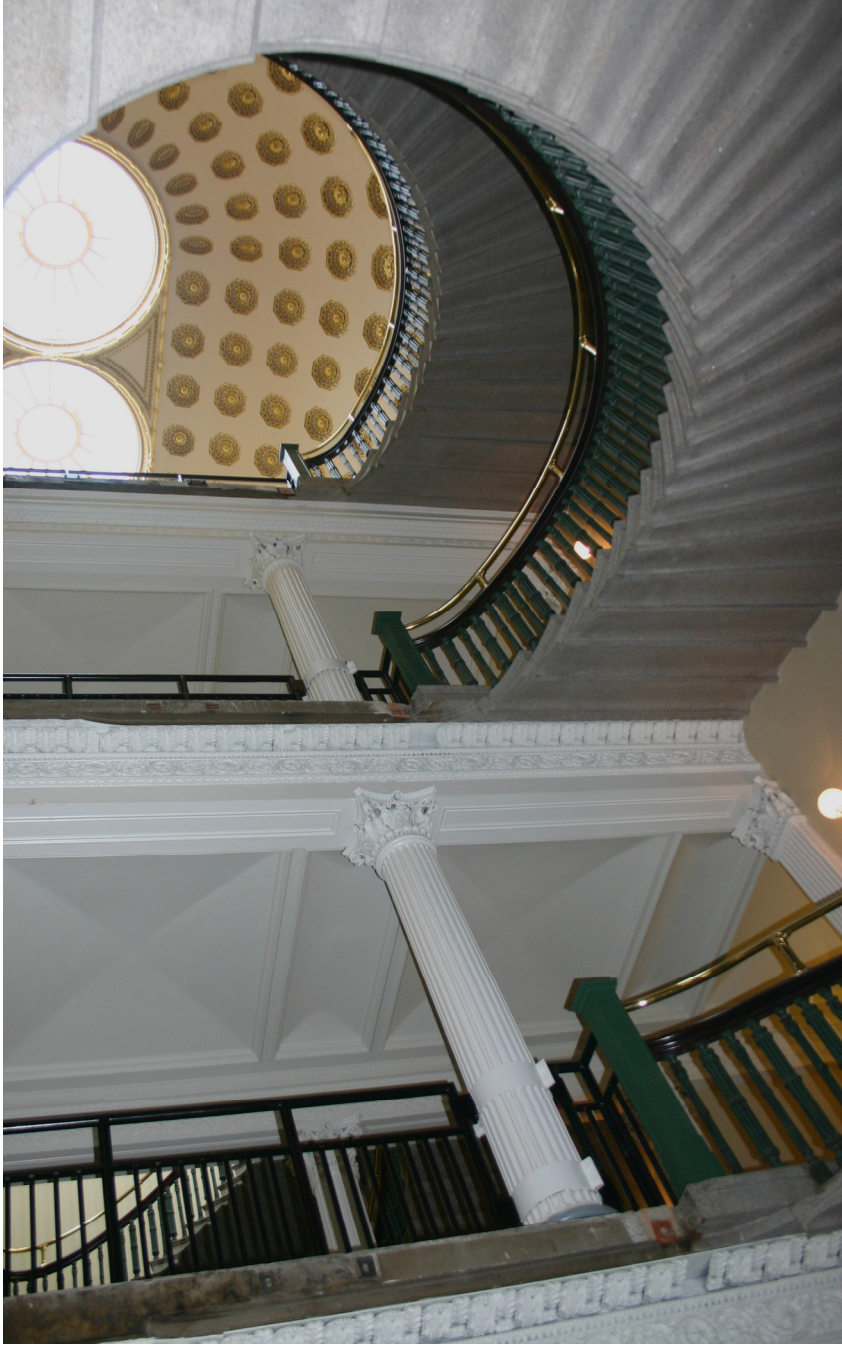
Figure 2, Treasury West Stair Balustrade Restoration, “Before”
