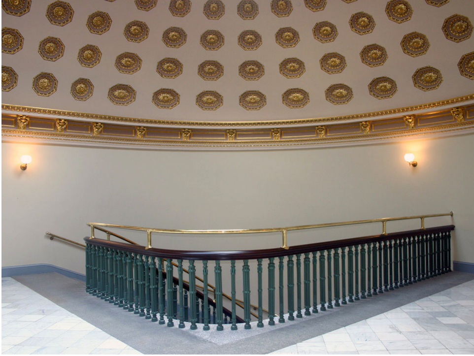
Figure 4, Treasury West Stair Balustrade Restoration, Detail
