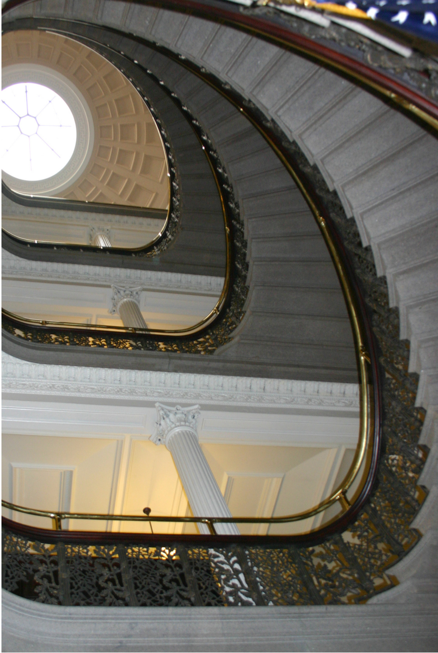
Figure 3, Treasury West Stair Balustrade Restoration, “After”
