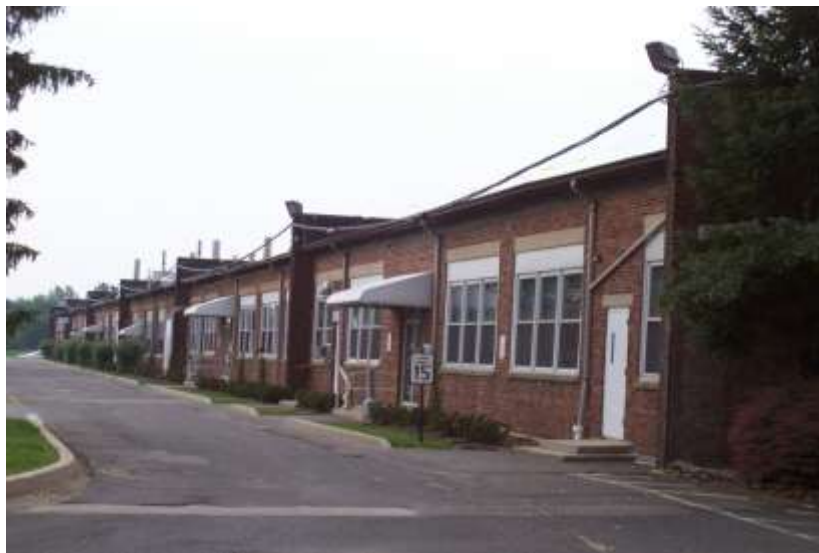
EPA's only National Register-eligible property, the Edison Environmental Center in Edison, New Jersey
