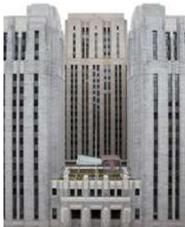
EPA Region 1 Office, Boston, Massachusetts
