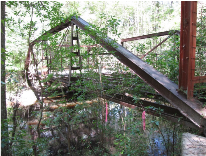
Iron Truss Bridge identified by Brockington and Associates during their ARPA permitted investigations at Carolina Sandhills. The abandoned span, though missing its wooden deck, appears to be in fair to good condition. It is similar to one in Pickens County, South Carolina that was built by the Greenville Steel Foundry Company in 1930.
