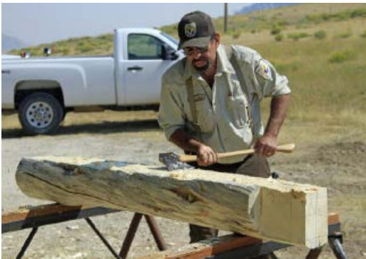
Figure 7: Fernando Escobedo hews the flat side of a log to fit against the backside of the wall's interior paneling.
