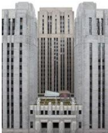
EPA Region 1 Office, Boston, Massachusetts
