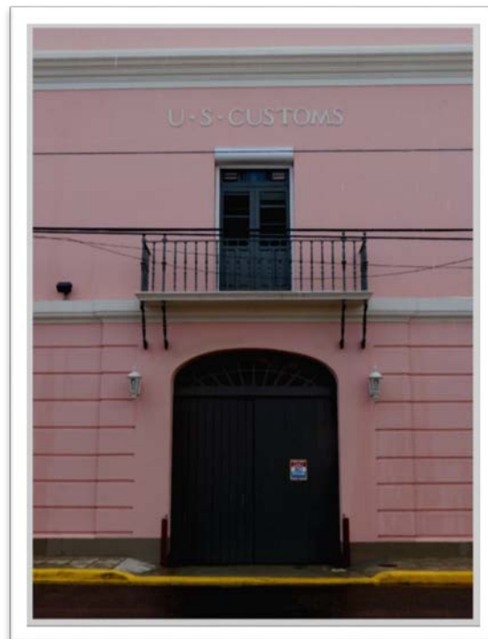
Figure 3.6. Door with Weir System to Mitigate Flooding and Window Hurricane Shutter.
