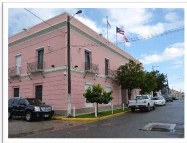
Figure 3.3. Ponce Customs House, Facing East.
