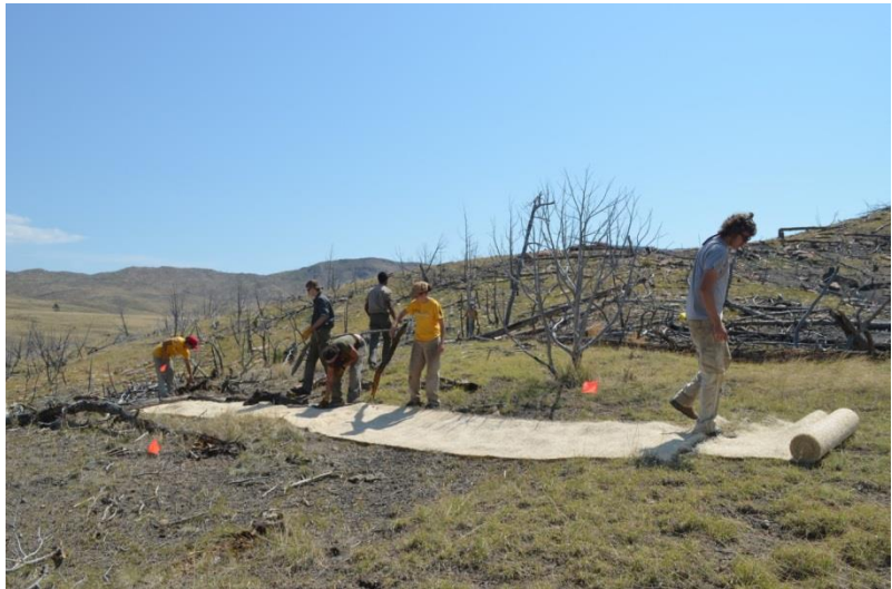
Figure 13. Corps team stabilizing soil erosion
