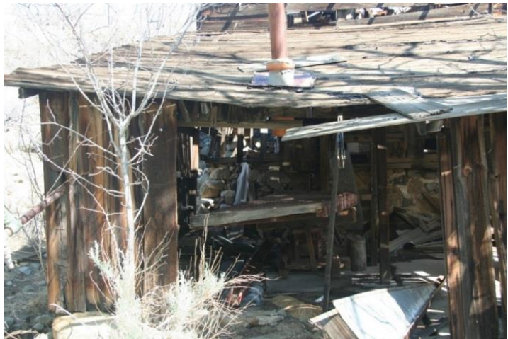
Figure 11. Cleveland Mill roof collapse imminent.
