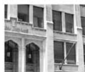
FIGURE 10 Exterior view of blast windows fabricated with custom muntins placing upper and lower panes in separate planes to simulate the appearance of double hung windows. (Mariah McGungie/GSA)
