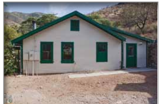
Florida Station Bunkhouse, before (2010) and after (2011) rehabilitation. Nonconforming siding has been removed to show original clapboard siding. (Photograph credit: Region 3.)
