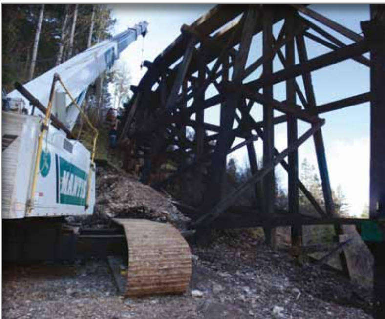
Stabilization of the Mexican Canyon Trestle using ARRA funds. (Photograph credit: Region 3.)
