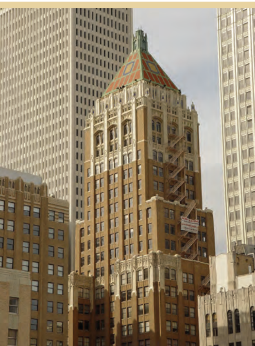
Historic rehabilitation project of the Philtower in downtown Tulsa, Oklahoma
