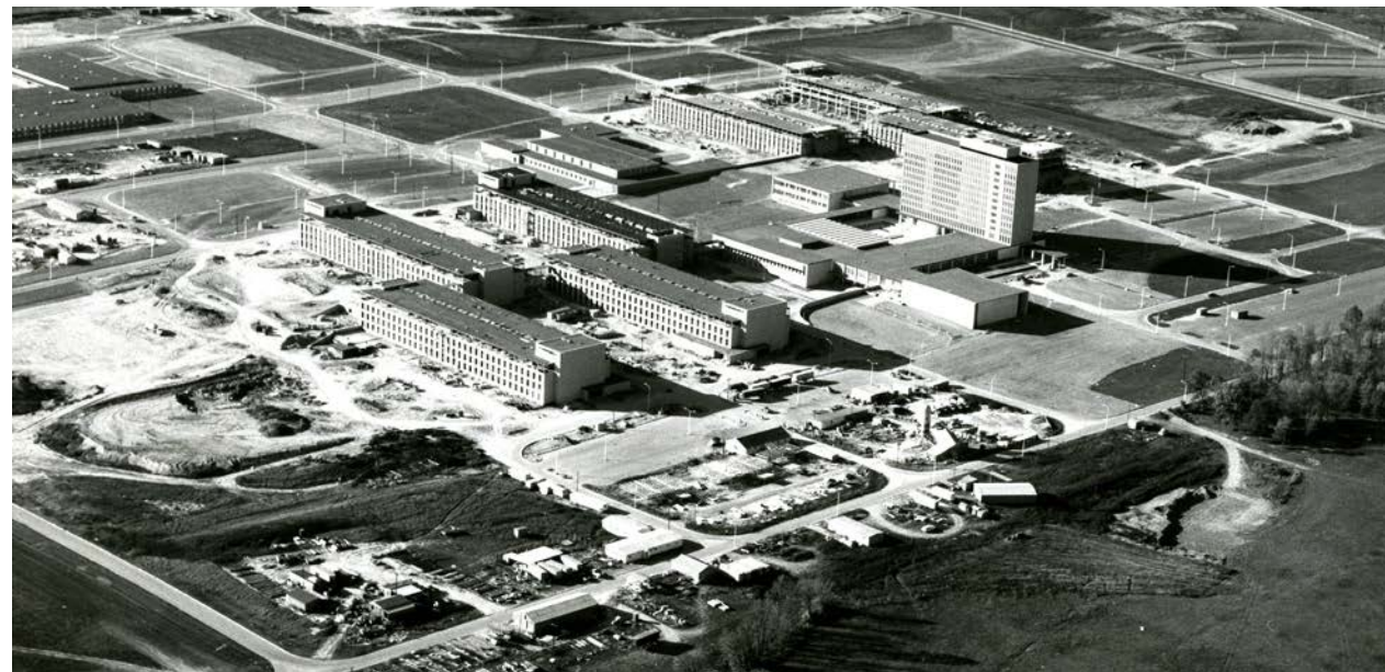
Aerial view of Gaithersburg campus construction in 1964 (NIST)
