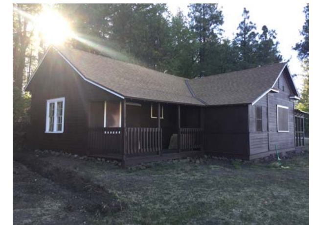
Mormon Lake Ranger House after rehabilitation (Jeremy Haines)
