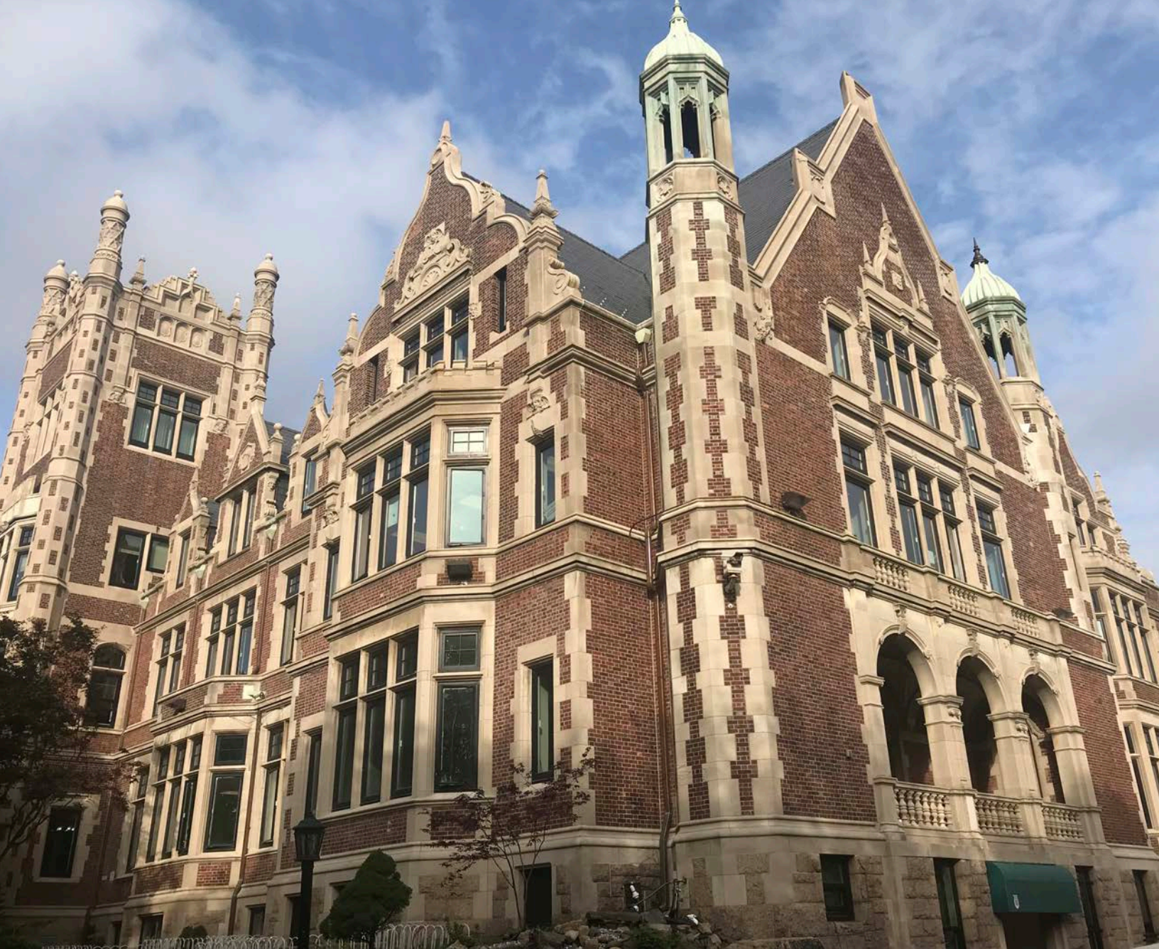
In 2017, the Department of Labor (DOL) completed a phased renovation of the Main Building (Building No. 1) at the South Bronx Job Corps Center, Bronx, NY. The work consisted of mechanical, electrical, and architectural upgrades throughout the building, and major restoration and renovation to the exterior façade. DOL worked closely with the New York SHPO to coordinate design and construction requirements in keeping with the historical integrity of the building. (DOL)
