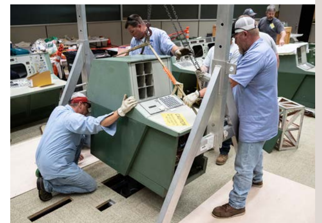
Installation of reproduced equipment. (NASA Johnson)
