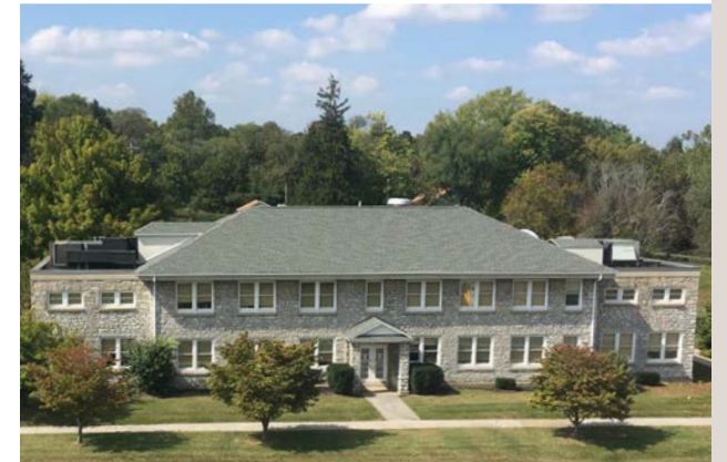
Front elevation of Leetown Administration Building (USGS)
