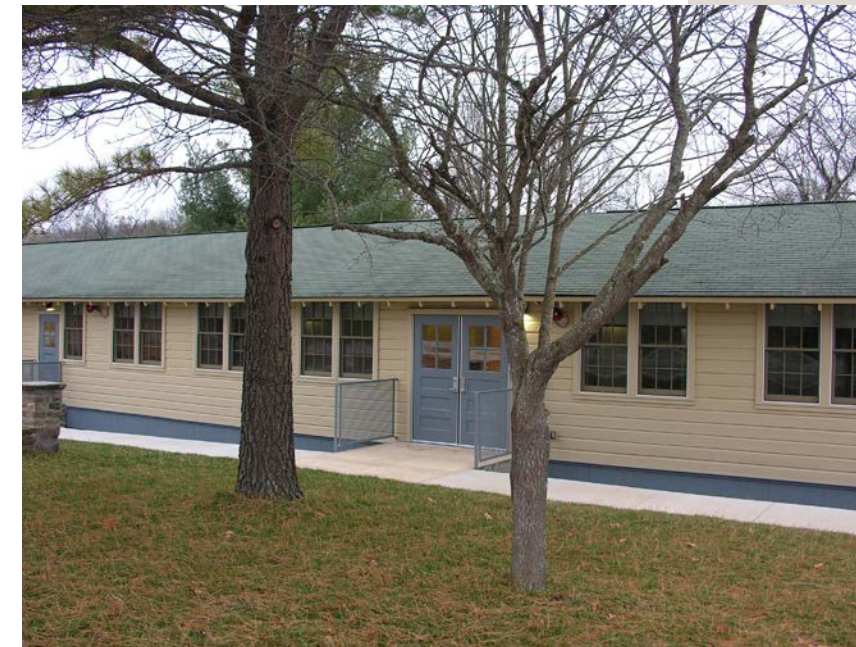
Countee Hall post-rehabilitation (U.S. Army)
