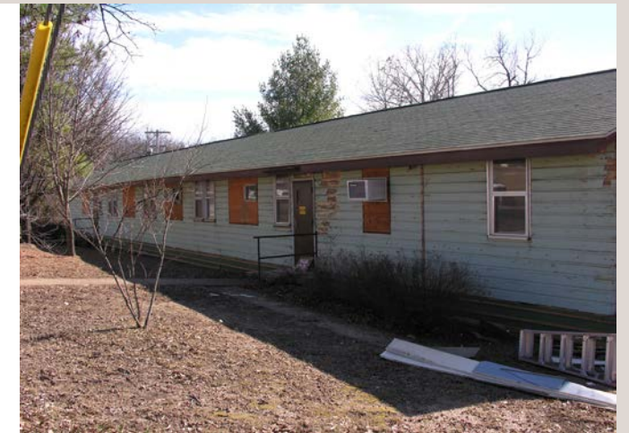
Countee Hall pre-rehabilitation (U.S. Army)
